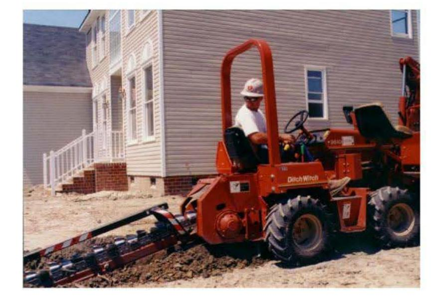
Figure 11: Typical Trenching Operation for Residential Services
